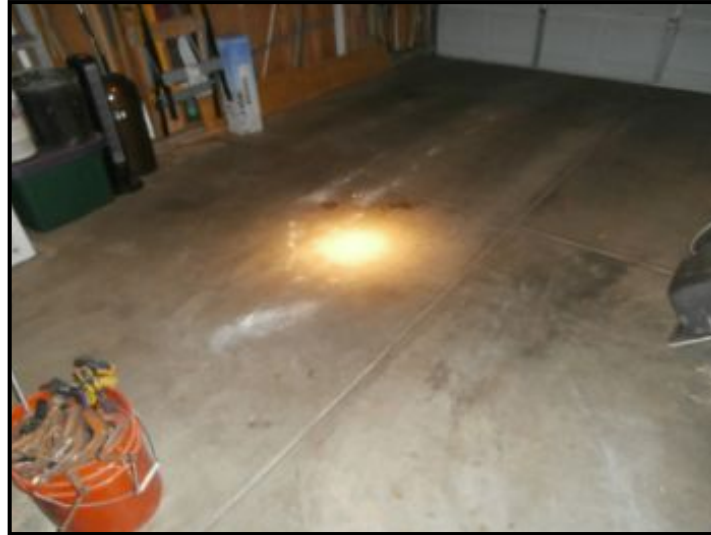
Floor in good condition
