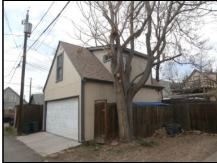
New roof - excellent condition.
