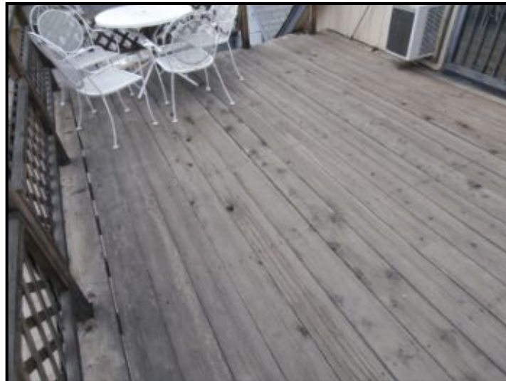
Upper deck off of master bedroom
