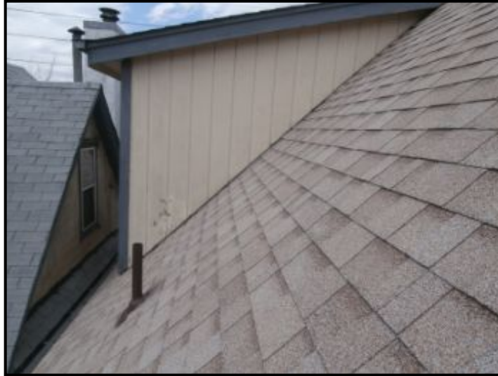
New Shingles - excellent condition
